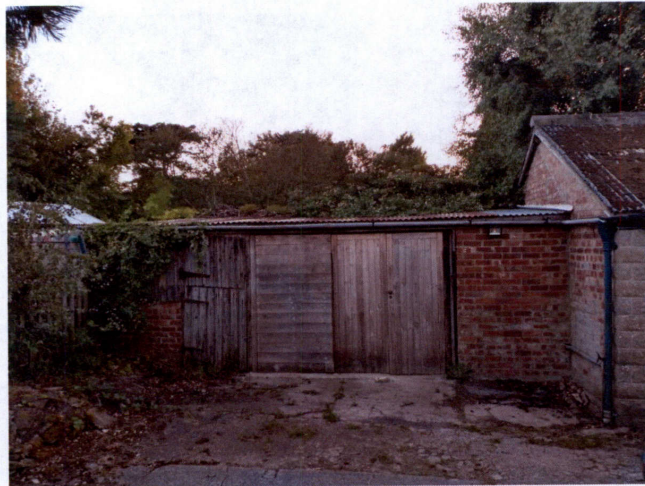
Image 04 - Side elevation of store building from the east
