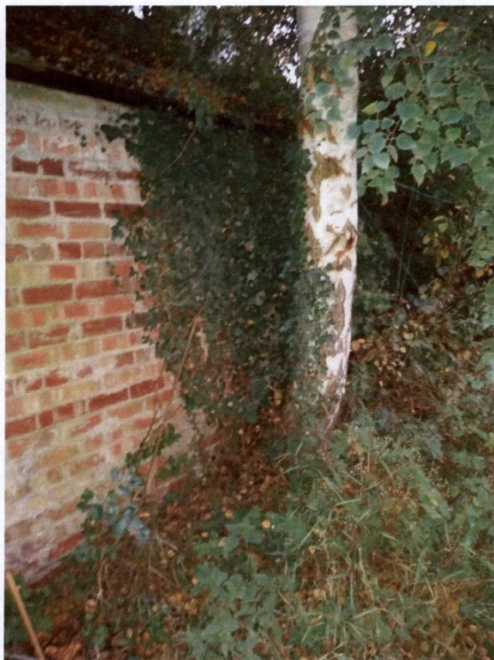
Image 07 - View of workshop brick wall from neighbour's side showing proximity of the birch tree to the building.
